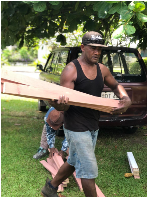
Prime mover ... Iosefo with timber for shutters at 23 Charlton Avenue
